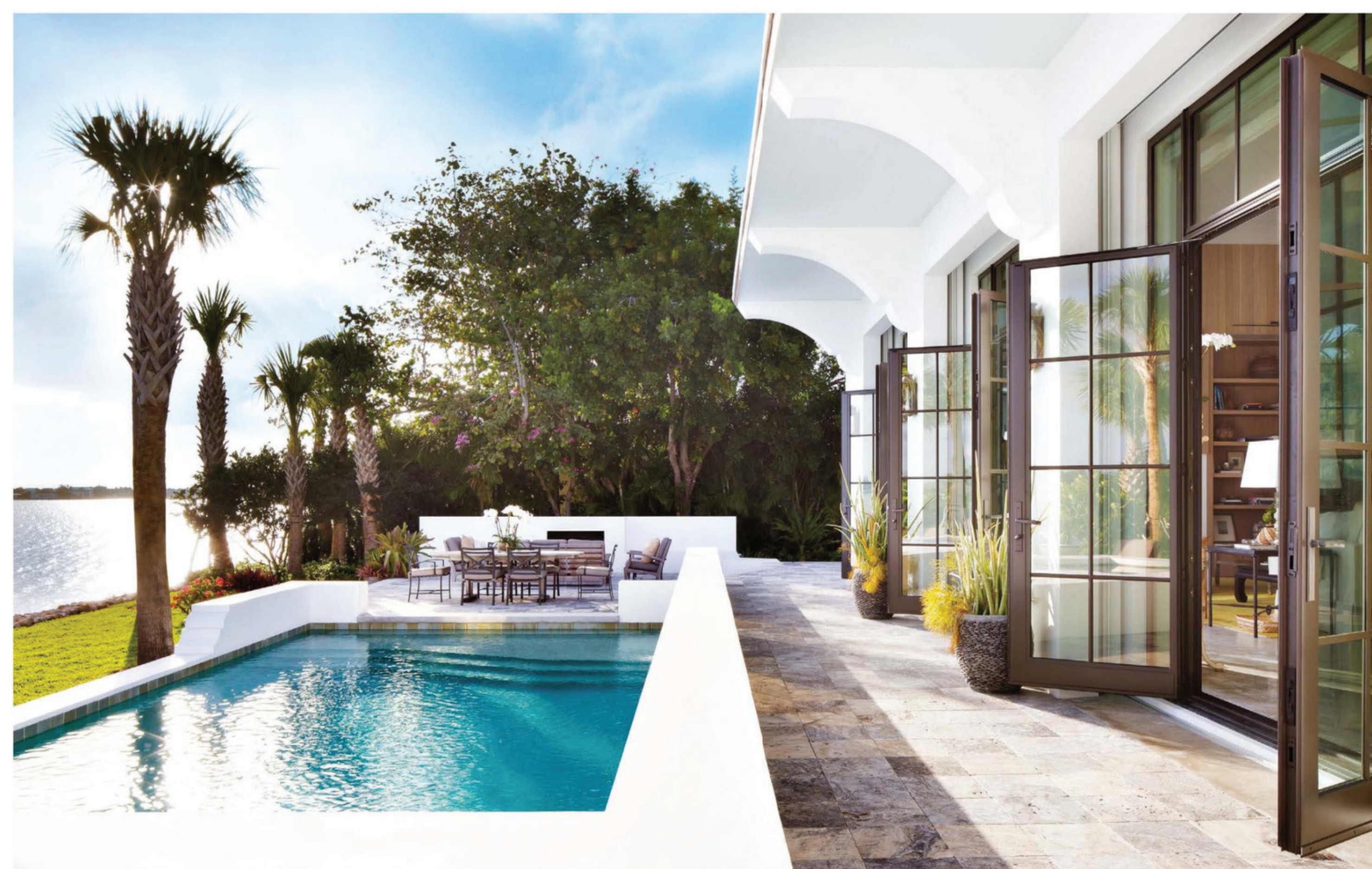
A 5-foot-deep eave, supported by simple concrete brackets, shades the south terrace overlooking the pool built by A & G Concrete Pools. Sabal palms, which keep views unobstructed, are planted on a grassy area that expands entertaining options. French doors by Hope's Windows were installed by WindowMan of South Florida.
